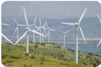
Air, Wind energy
