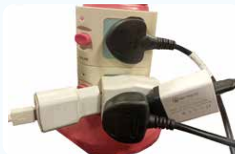
Overloaded plug sockets can damage the household electricity supply and cause a fire
